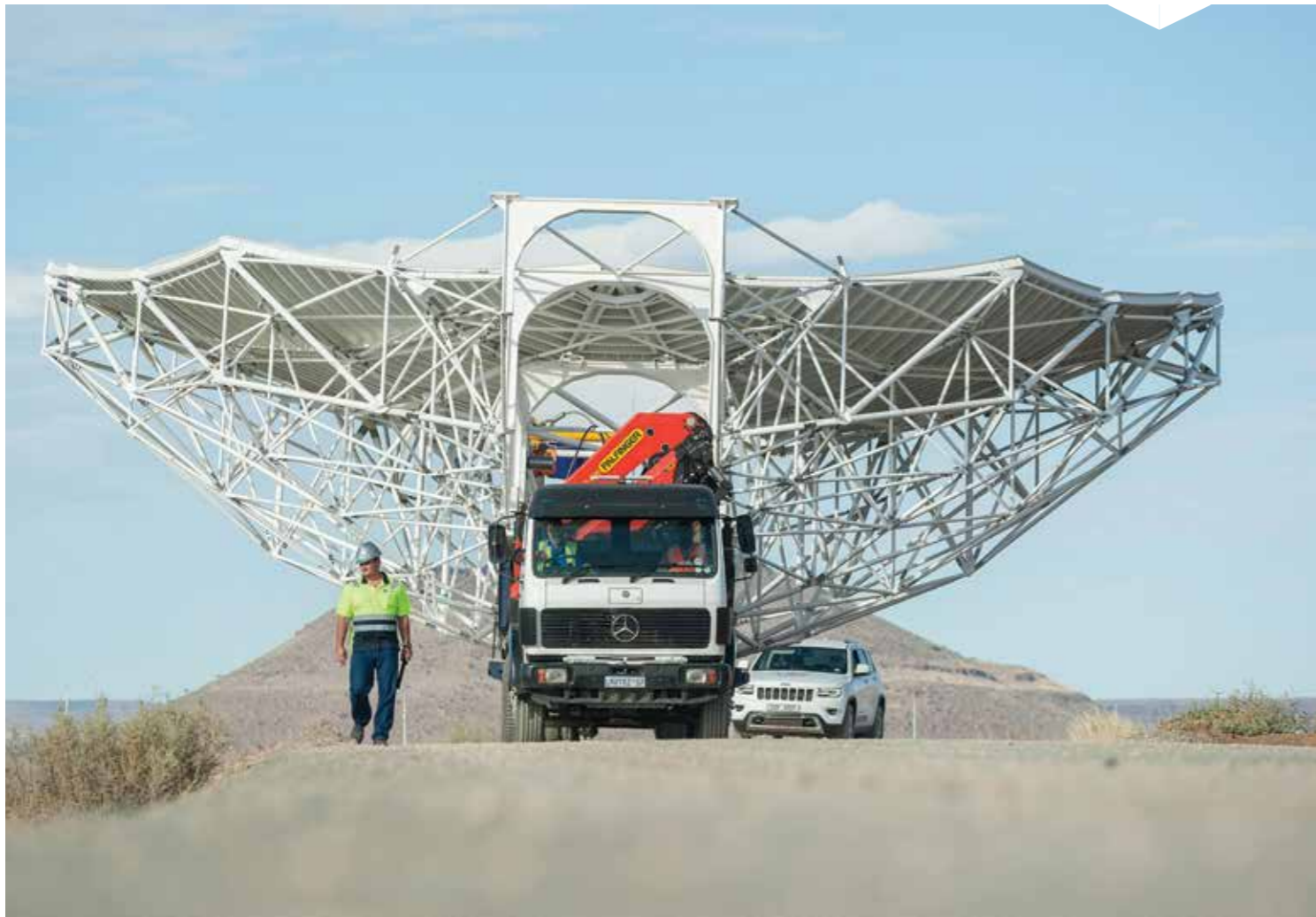
The construction of MeerKAT antenna. Image courtesy of SKA South Africa.
